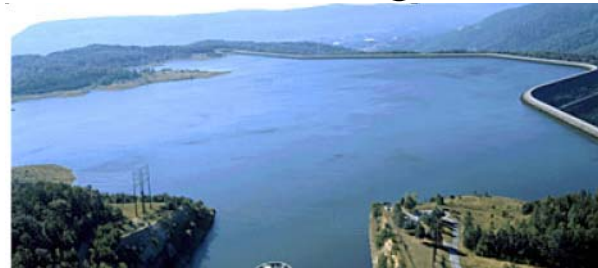
The Raccoon Mountain project is TVA's largest hydro facility. Water is pumped to this mountaintop reservoir and then released to generate electricity when added power is needed by the TVA system.
